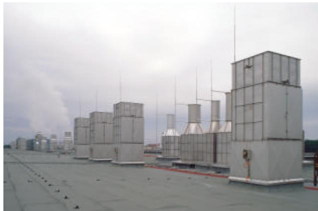
Figure 6. Silencers on the building roof, Haindl Papier Augsburg PM3.
